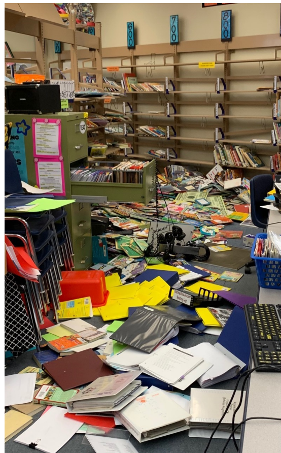
After the Ridgecrest California Earthquakes in 2019, even undamaged buildings sustained significant content damage.
